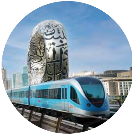
Dubai Metro (Red & Green Lines) Construction of the fully automated, driverless metro system including viaducts, tunnels, and 47 stations
