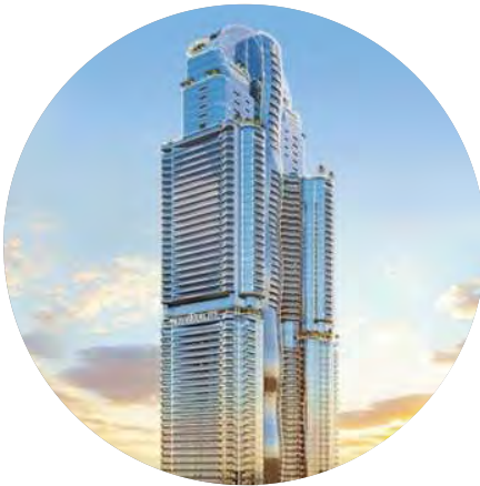
Al Habtoor Tower Construction of a 82-storey residential tower within Al Habtoor City
