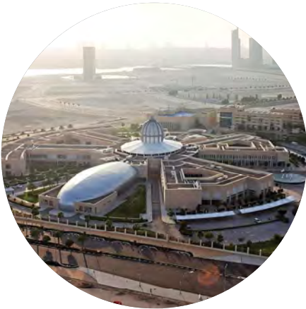
Sorbonne University Abu Dhabi Construction and completion of an educational facility comprising academic and non-academic buildings
