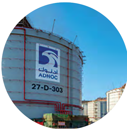
Fuel Storage & Distribution Tanks Construction of fuel storage and distribution facilities including pipelines and pumping systems
